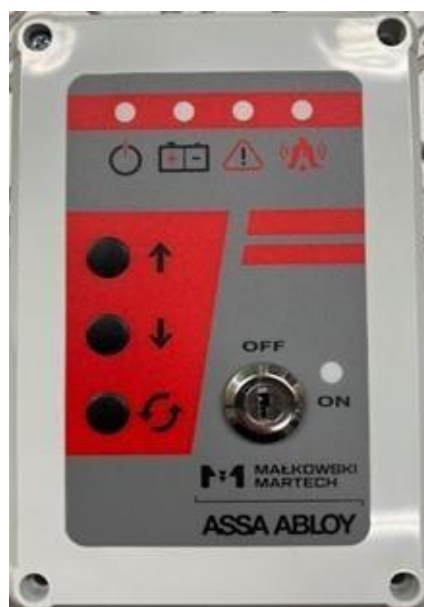
Drawing 1. Fire protection curtain gate key switch.
